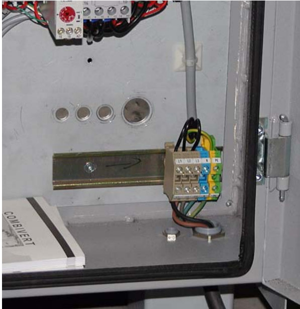
Fig. 5-39: Mains connection
